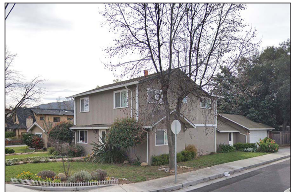
Nearby two-story house on Fisher Avenue
