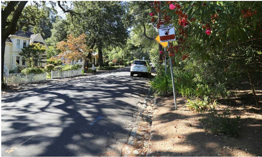
Photo 4: Looking south on Chestnut Avenue from the approximate location of the driveway if located 50 feet south of the intersection.
