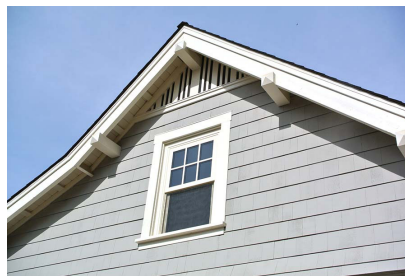
Gable end beam ends and vent detail
