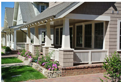
Porch columns, bases, caps, beams and railings
